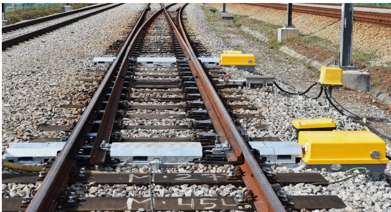
Turnout controlled by two EP-6xx
